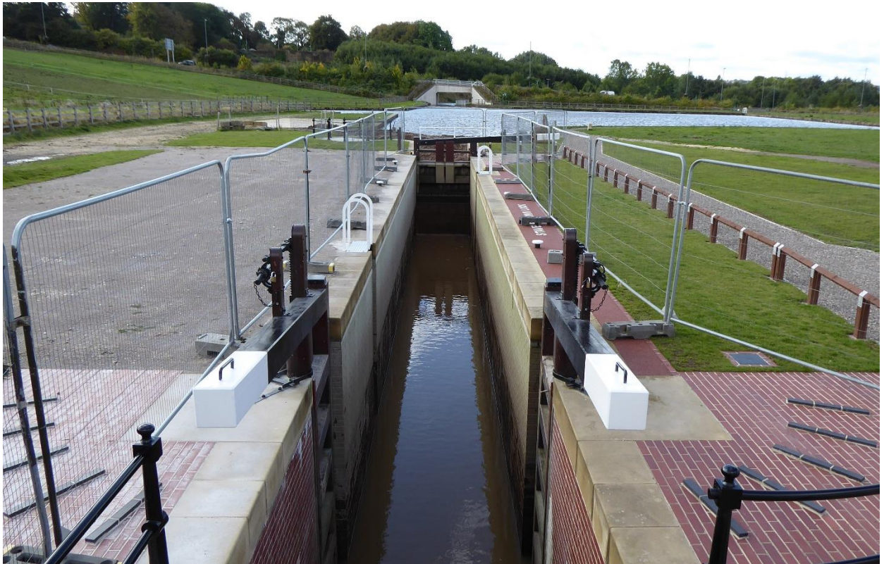
Figure 6.2: Staveley Town Lock (No. 5a), at Staveley Basin. Eckington Road Lock (No. 5b) and Railway Lock (No. 5c) will be similar in construction and appearance
