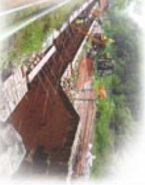
Building Dixon's Lock No 4 at Brimington
